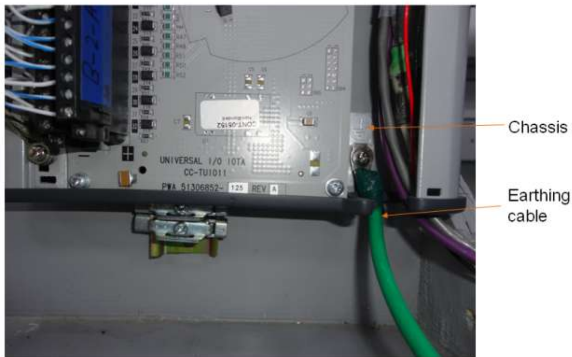
Figure 164: Grounding connections
