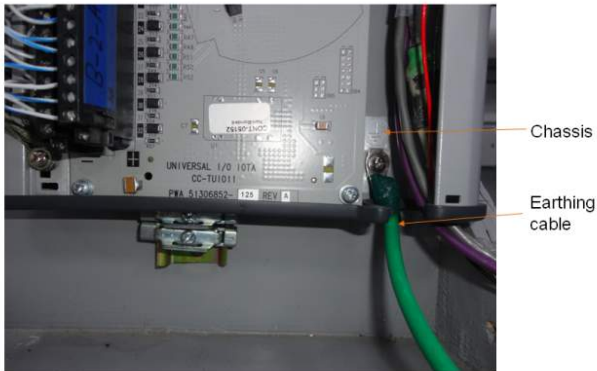
Figure 164: Grounding connections
